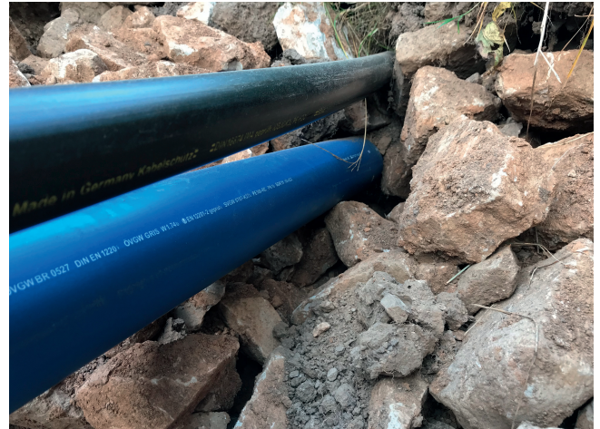
Fig. 4. Trenchless pipe laying is less energy and work intensive than conventional methods. It is also suitable for installing high-voltage power cables, e.g. during the change in energy distribution to decentralized supplies. © Gerodur MPM Kunststoffverarbeitung
